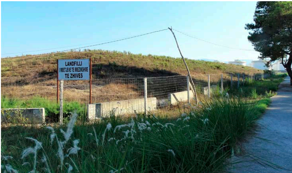
Figure III-3.11 Above: The sewage dumping of black waters into the canal that crosses the Soda Forest. Below: The authorised dump for mercury wastes. In the background the Petrolifera Italo-Albanese plant.
