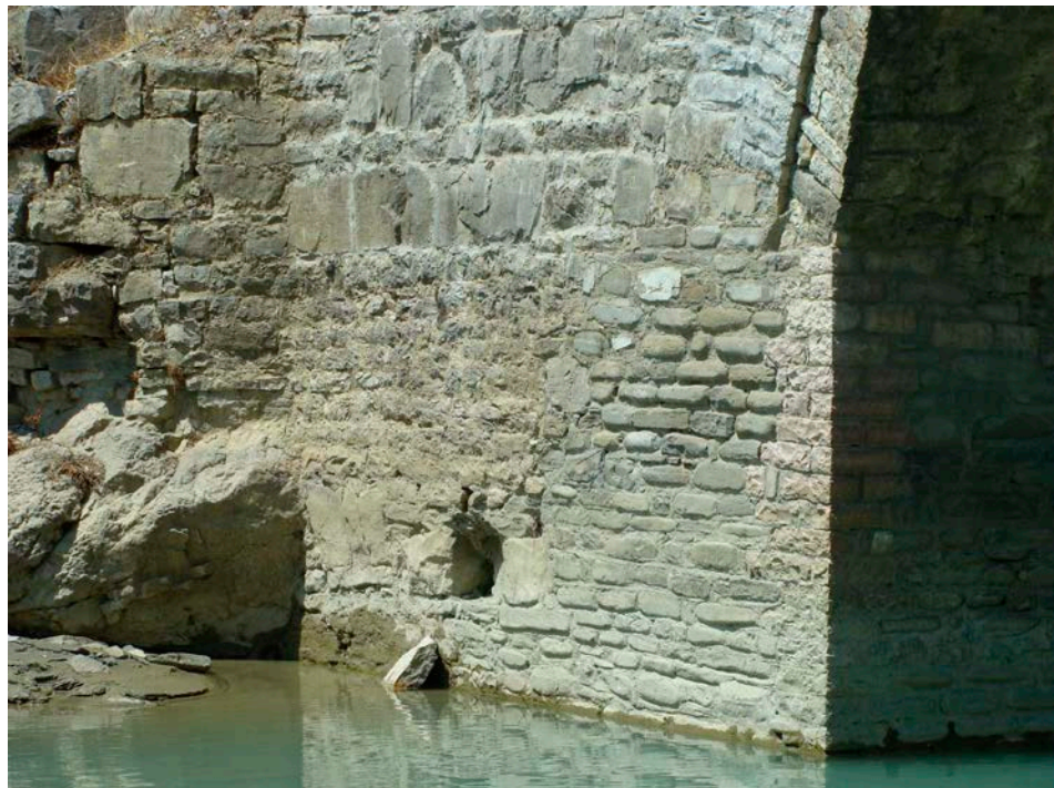
Figure I-5.1.6 – A detail of the abutment restored in 1982.
