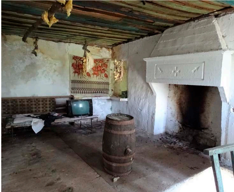
Figure II-4-11 The interior of a traditional dwelling with a wooden false ceiling and a widespread type of fireplace.
