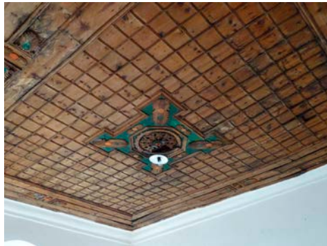
Figure I-4.1.11 A decorated wooden false ceiling in a guest room.
