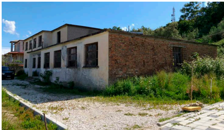
Figure III-4.4 The former village school, abandoned since 2007.
