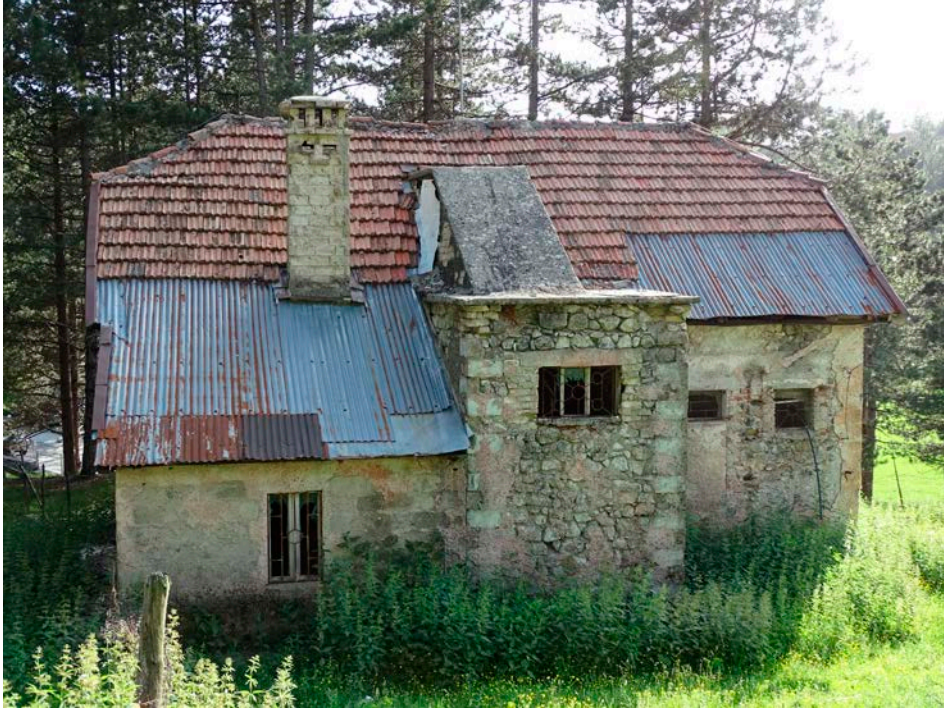
Figure II-5.8 An example of the additions and transformations that occurred over time on the rear facade of a villa.
