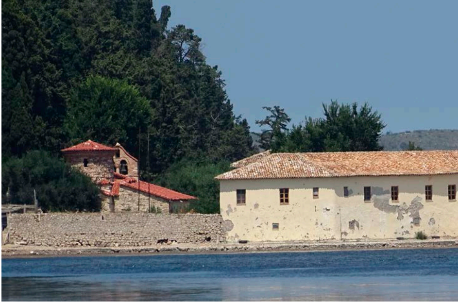
Figure III-5.9 A view that highlights the chromatic difference between the roof covering of the church and that of the lodgings.
